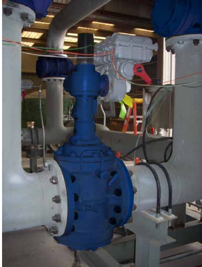
OmniSeal® DBB expanding plug valves during installation
