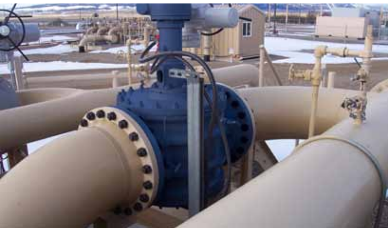
OmniSeal® DBB expanding plug valves in service
