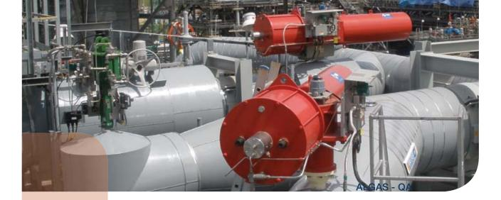
Quick acting pneumatic, hydraulic, electro-hydraulic actuators
