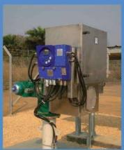
The ITVC is the electronic logic controller which can control and activate the main HPU functions (LOCAL / REMOTE OPERATION, ESD FUNCTION, MOTOR/PUMP CONTROL, MONITORS OPERATING PRESSURE AND OIL LEVEL, DIAGNOSTICS, ACTUATOR Solenoid Valve coil test every 8 hour as per the latest requirements of IEC-61508 to achieve SIL 3).
